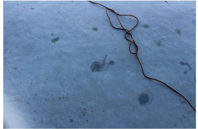
Figure oB-00060a – Pool Floor with Nodules Over Cracks and Sub-Surface Trapped Water
