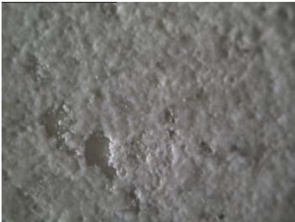
Figure 19 – Aggregate Exposure of Lightly Etched Plaster
