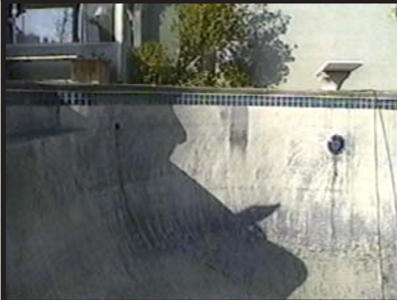
oB-00005Dh – View of deep end walls
