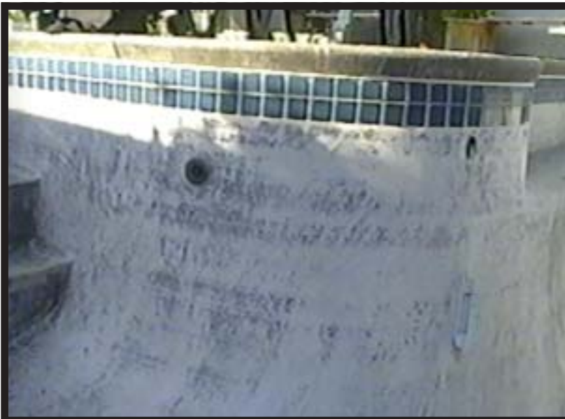
oB-00005Dg – Horizontal water lines and bottom-to-top trowel pattern
