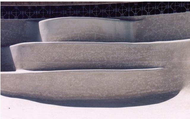
Plaster soft spots are surface blemishes that are caused by a combination of plastering errors. These include the over-use of calcium chloride set accelerant, and (as subsequent coping techniques) late over-troweling and adding water to the surface during late troweling.
